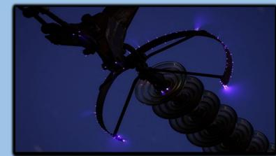
Figure 1: Glow Coronas form on the edges of a powerline transformer (Berkoff, 2005).
